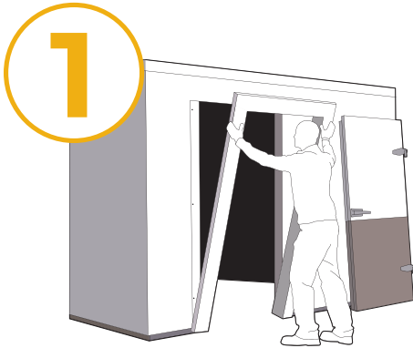
1 Set the replacement frame in place.
